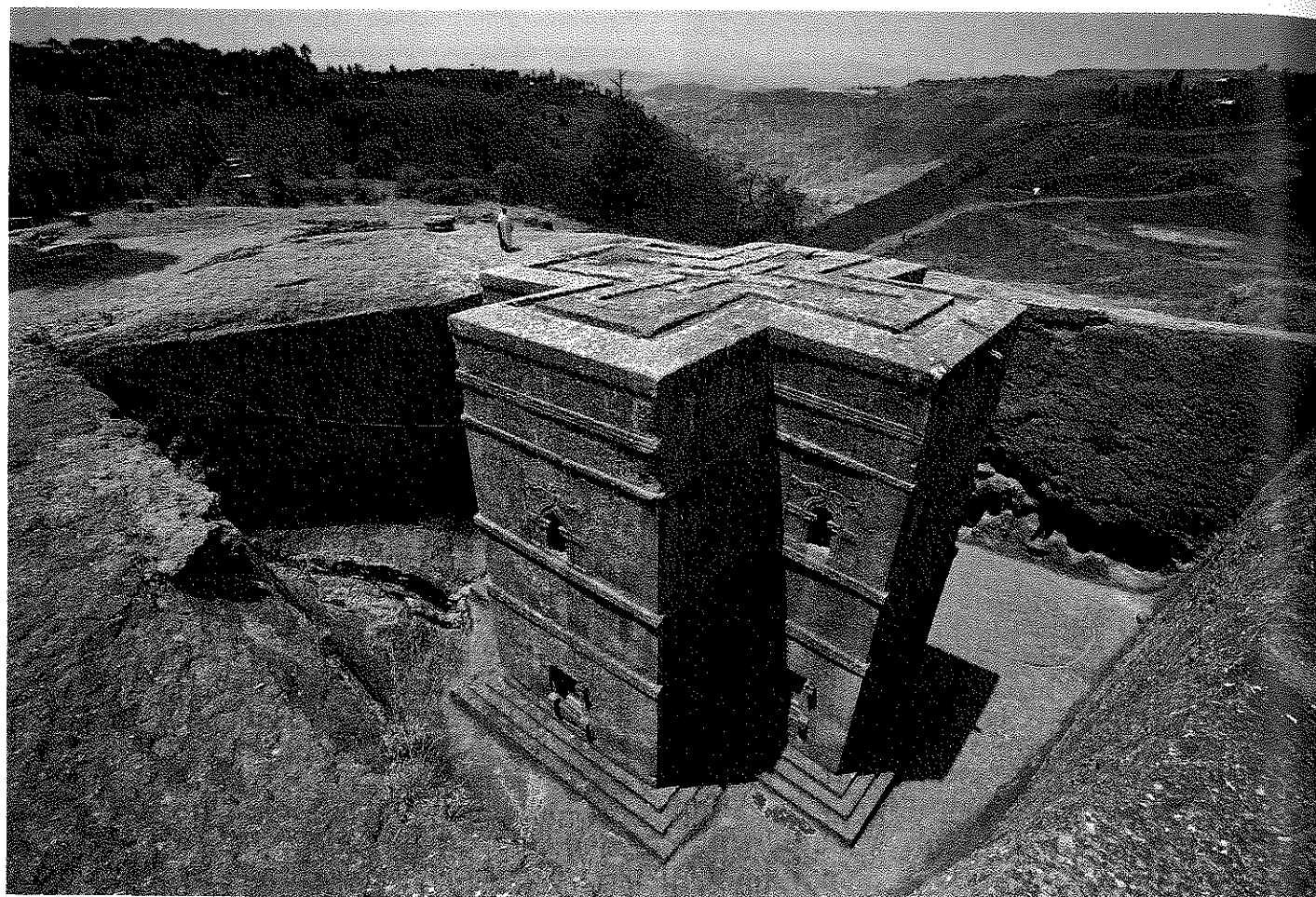
The church of St. George at Lalibela, Ethiopia, a massive structure in the form of a cross. Workers excavated the surrounding earth and then carved the church itself out of a rock.
